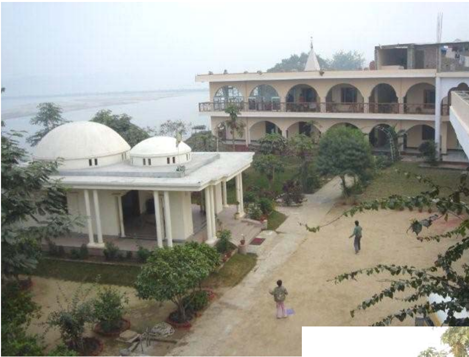
A view of the facility and the beginnings of a new color for the buildings.
