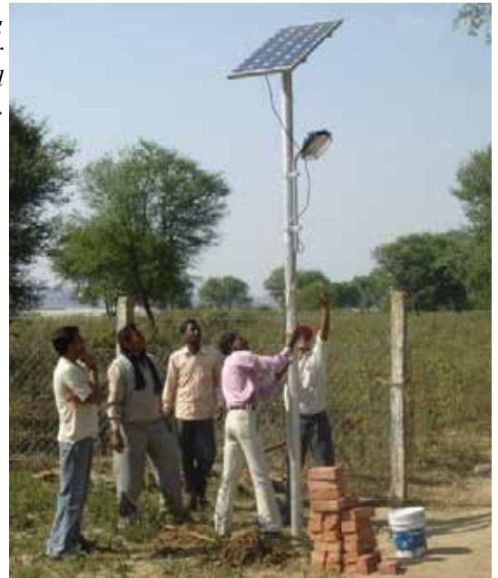
Installing solar powered street light.
