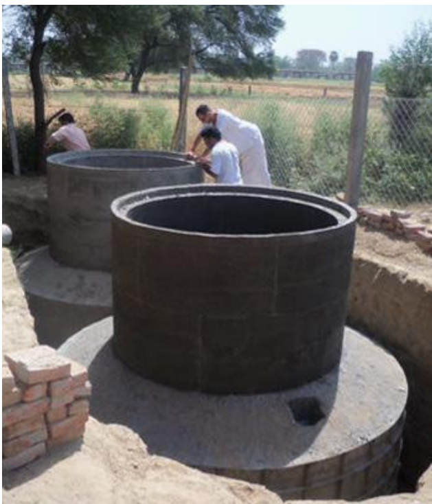
Nearly complete bio-gas system.
